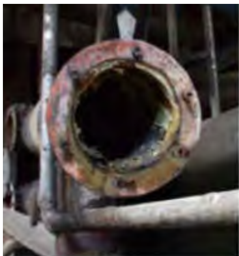
Metal pipe shown here exhibiting both internal and external corrosion.
